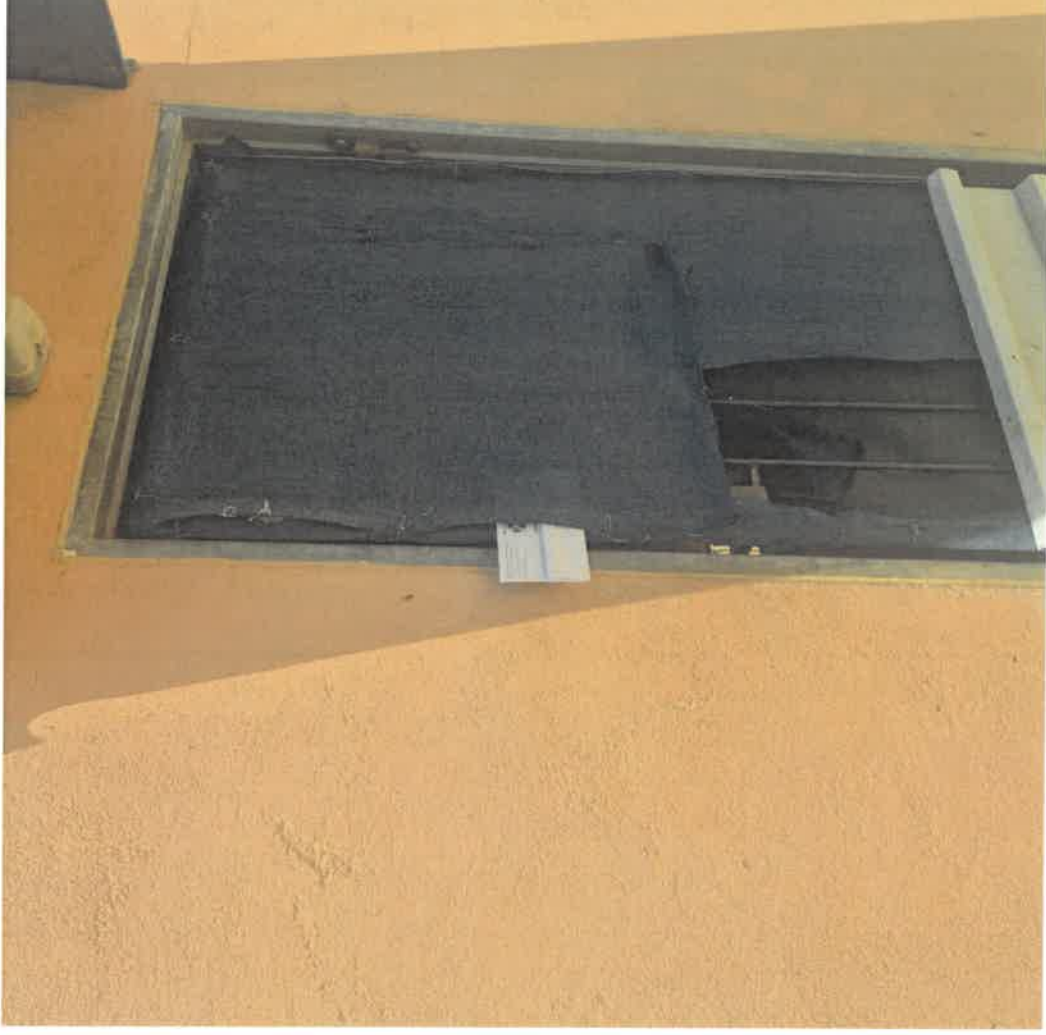
Photo 5 - Warning notice attached to the door
